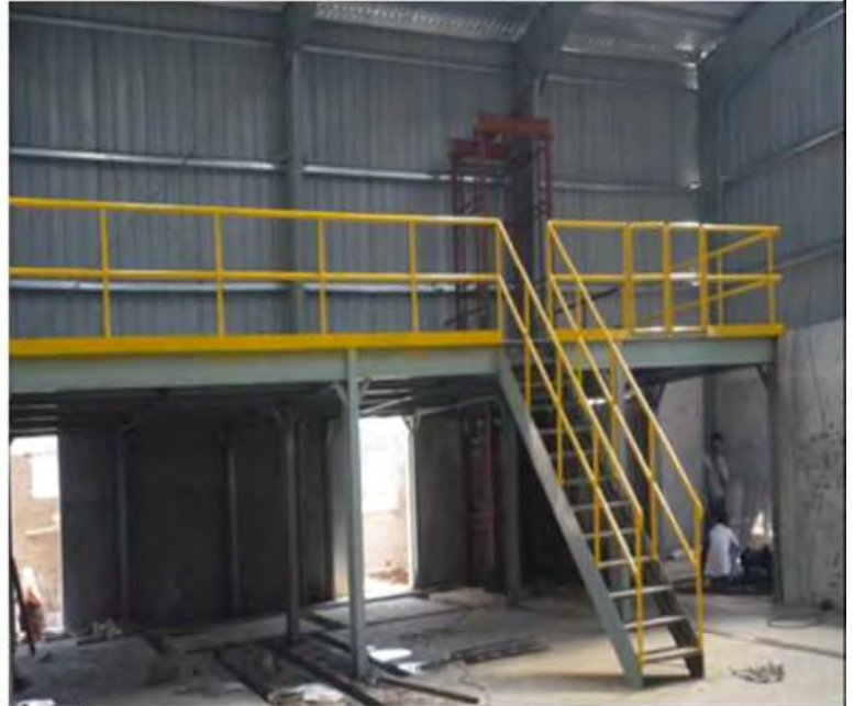
Welded Mezzanine Floor
